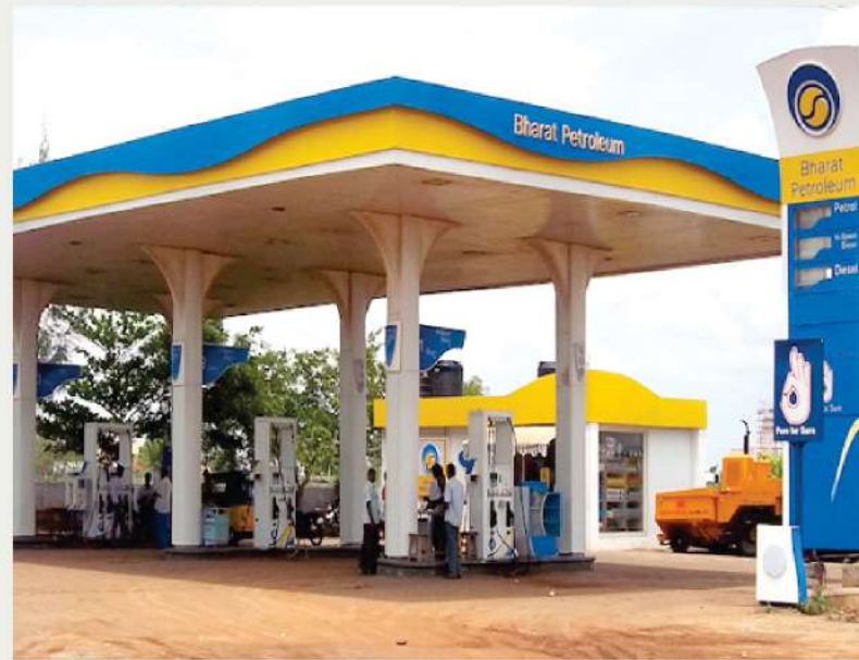
Bharat Petroleum Corporation Ltd
