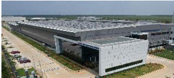
AIR CONDITIONING MANUFACTURING UNIT At Sri City Andhra Pradesh
