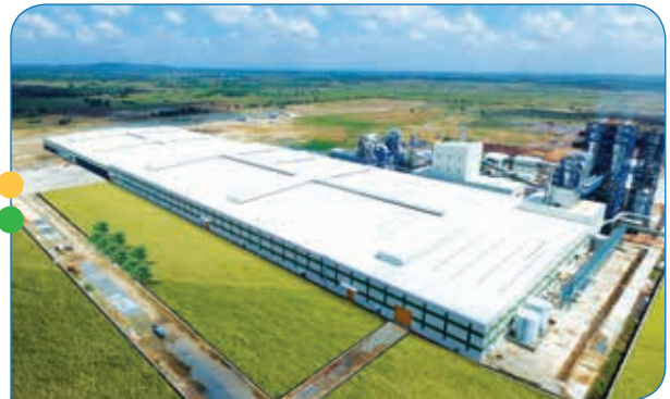
Greenpanel Industries Limited, Chittoor
