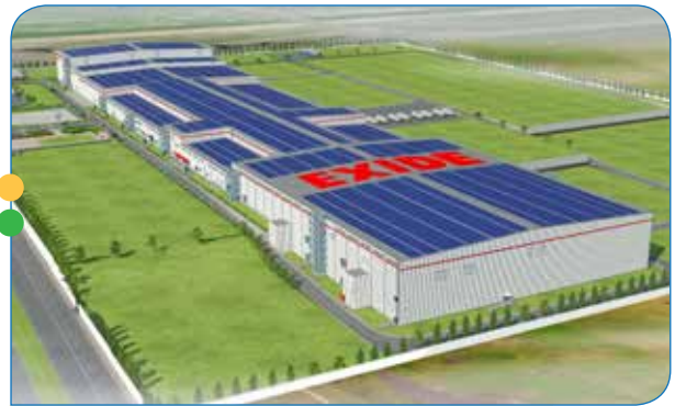
Exide Energy Solutions Limited, Bengaluru
