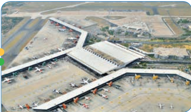
Indira Gandhi International Airport Terminal 3, New Delhi
