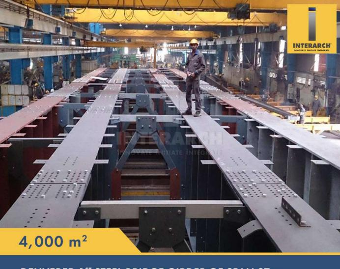
DELIVERED 1<sup>ST</sup> STEEL BRIDGE GIRDER OF SPAN 37m DELHI METRO RAIL CORPORATION LTD BRIDGE GIRDER
