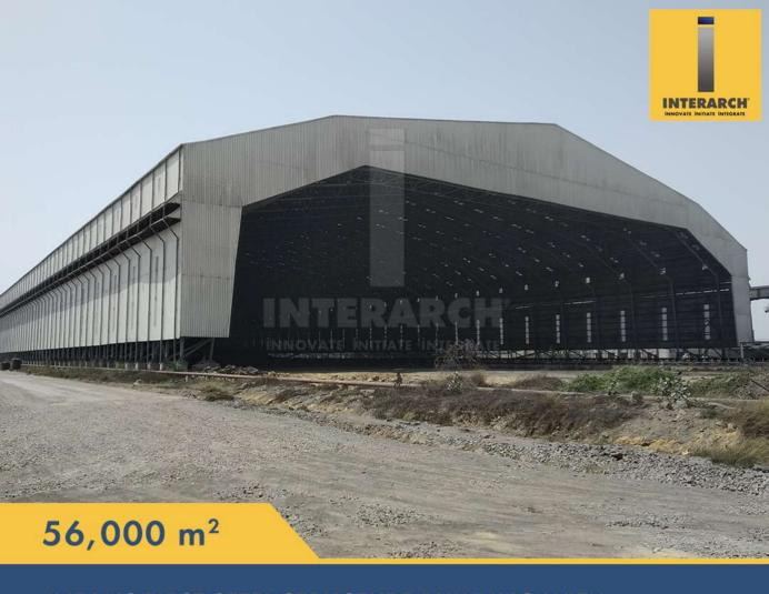
INDIA'S FIRST STEEL STRUCTURE BUILDING WITH A CLEAR SPAN OF 120m
