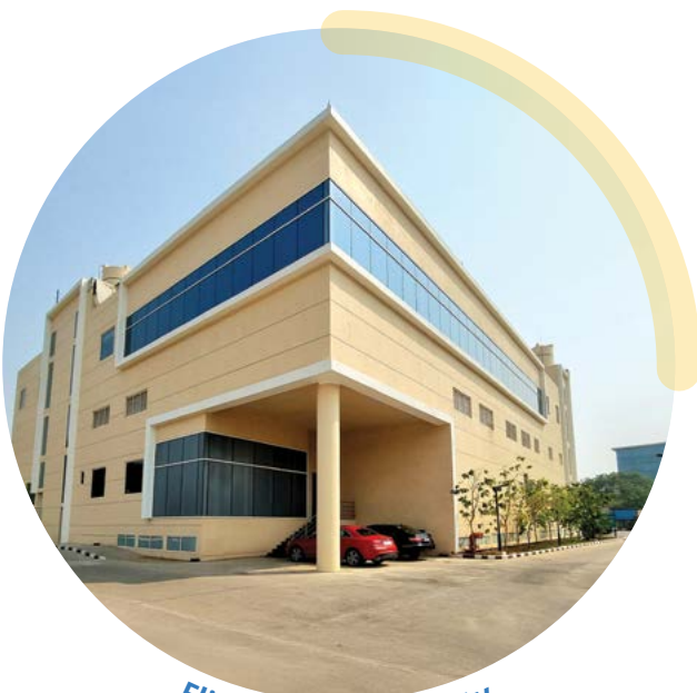
Flight Kitchen Facility
