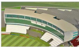
Interarch has to detail the structure of 23 m wide and 125 m arc length with tubular truss structure at a height of 53.00m from Ground level. Complicated truss system with lot of splice connections has been detailed with latest software TEKLA and accuracy maintained with 3-D model. It has primary & secondary trusses which is 100% Pre-fabricated at a factory in controlled quality standards, transported and bolted at a given heights as per Interarch's EHS Policy
