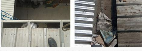
2. Roof inspection should be done to check for any damages to roof sheets, flashings etc. due to winds, man movement or animals etc.
