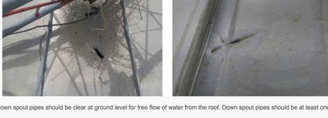
3. Opening of all down spout pipes should be clear at ground level for free flow of water from the roof. Down spout pipes should be at least one foot above the ground level
