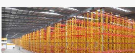
The total project consumed more than 2700 MT of steel for structural system and over 1, 65,141 Sq. M. of roofing & sheeting was supplied and installed. The buildings were manufactured in Interarch Pant Nagar Plants
