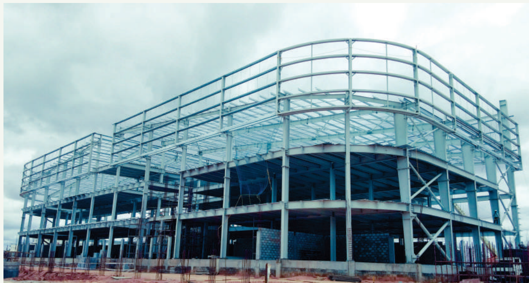
Typical Primary and Secondary Framing Systems
