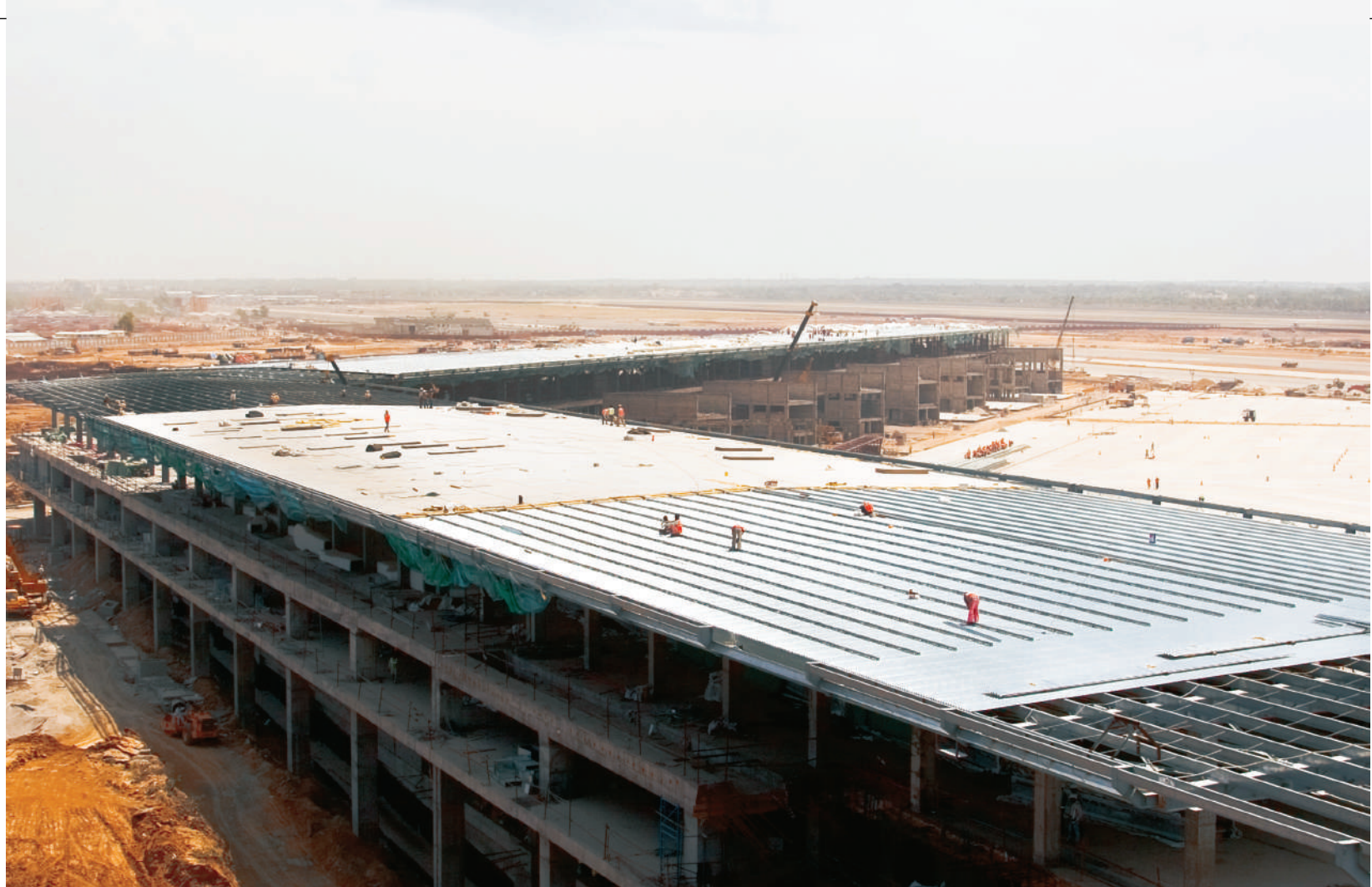
Standing Seam Roofing System - IGI Airport Terminal 3, PIERS
